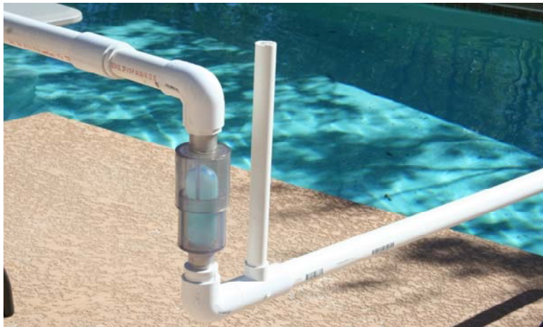
Figure 9 Installation of a Vertical Vent Pipe installed directly downstream of a P-Series Air-Trap to prevent a suction pressure from developing below the trap. A suction pressure could develop depending upon the length of drainpipe, the diameter, and the water flow rate.
