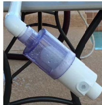
Figure 5 P-SERIES Air-Trap installed at 45° angle can reduce trap height by 30% and operate at up to 5" of positive pressure.
