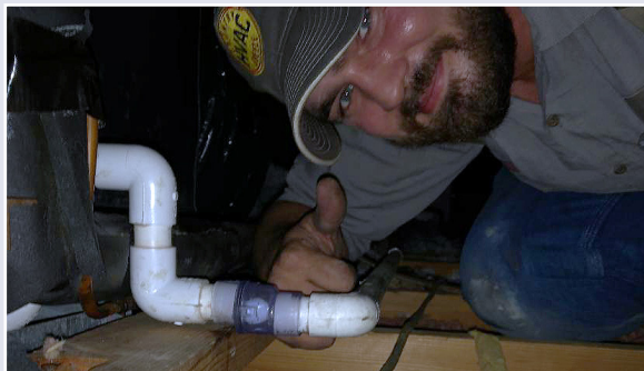
FCN-Series indoor residential attic install, negative pressure orientation. Tight space no problem, all thumbs up from the technician!
