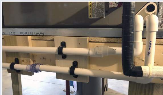
FCN-Series negative pressure commercial installation, an Air-Trap on both the main condensate drain pan line and secondary pan line.
