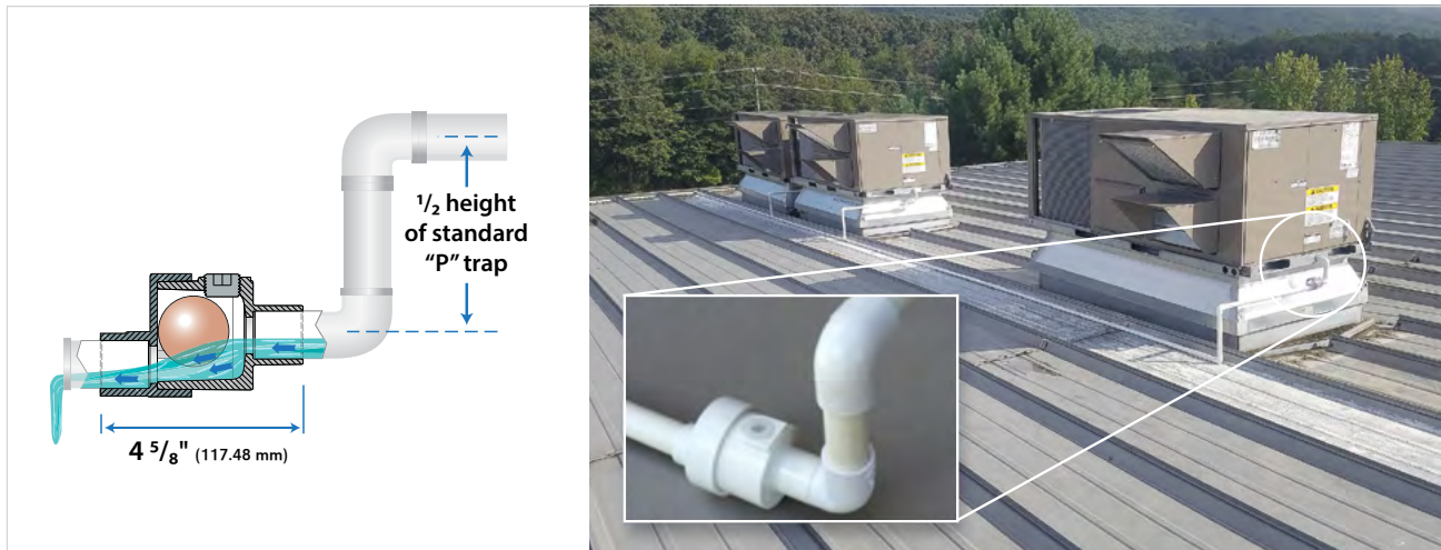
Figure 7: Des Champs HVAC Air-Trap RLC-Series
